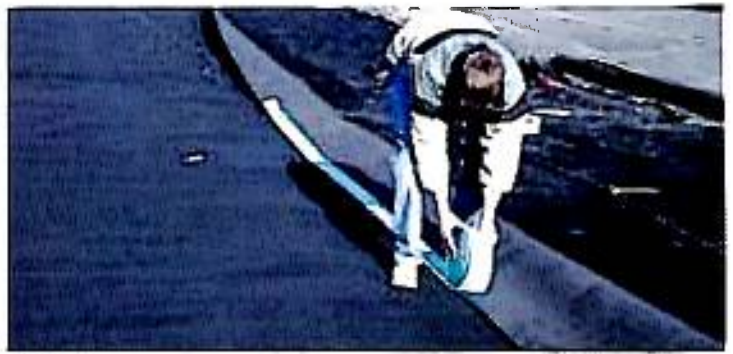
Figure 4: Reinforcements of Roads
